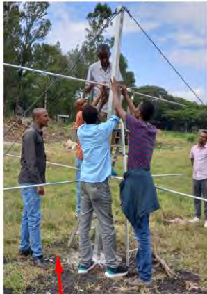
PhD students assembled Meteor Radar antenna at Bahir Dar University
