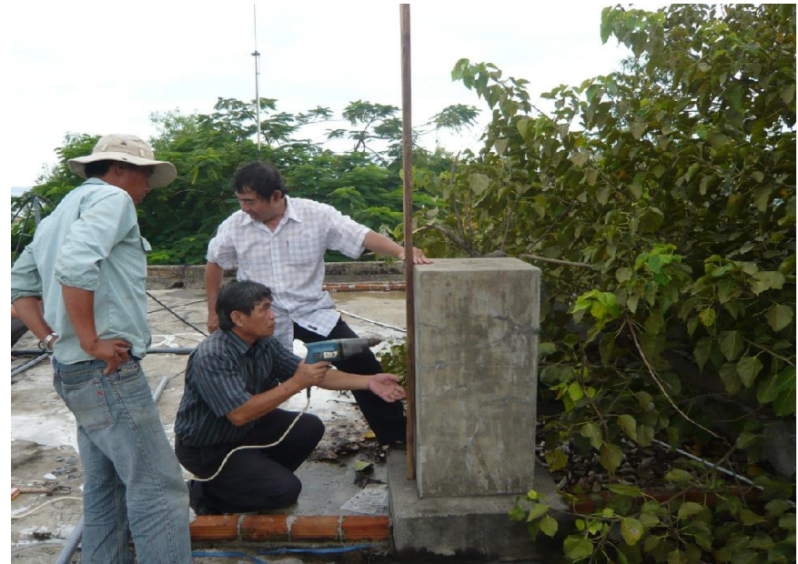
Setting up the GPS antenna
