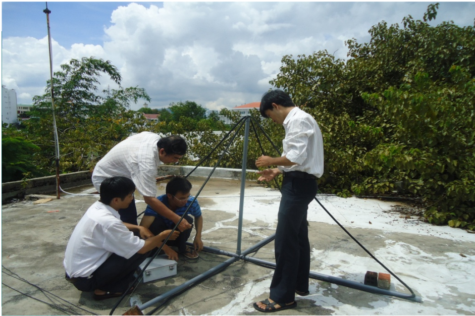
Assembly the VLF Antenna
