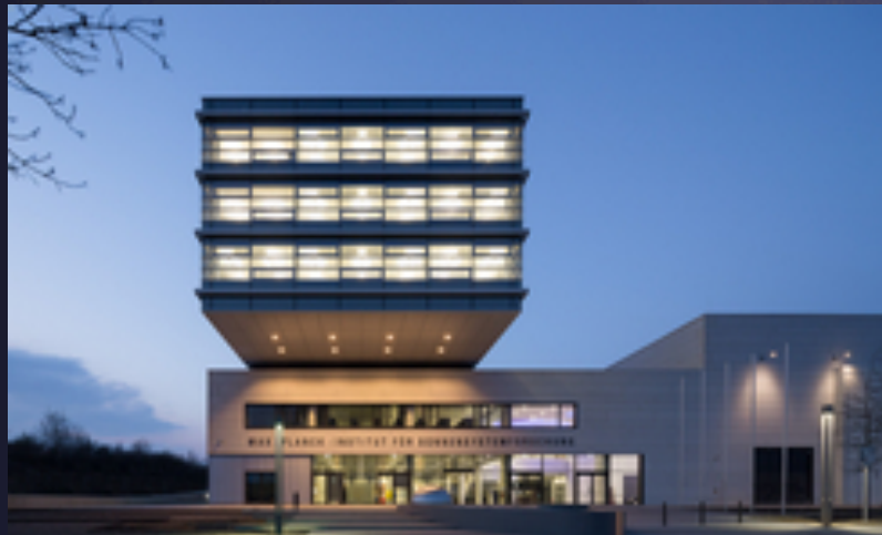
Brand new MPS building in Göttingen
