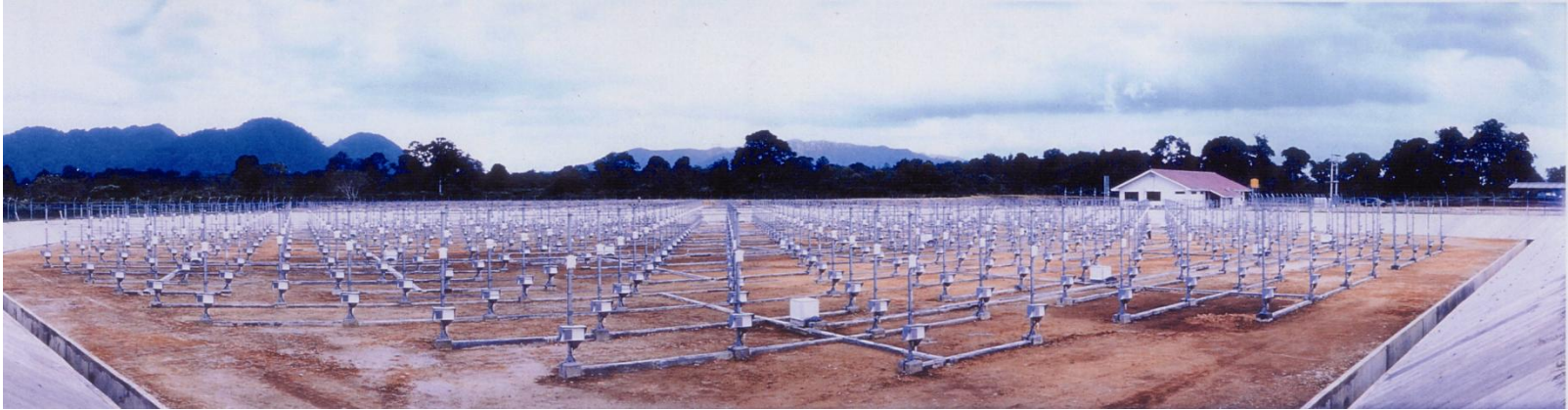
Antenna field (110m in diameter)
