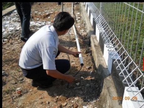
Passing the cable through the orange tube
