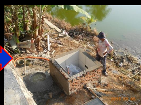
Orange tube after being buried
