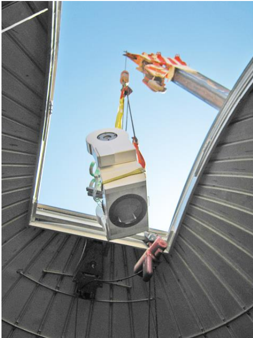
Photo 2: Carrying the fork-mount of the FMT in the astrodome (Dec 2014)
