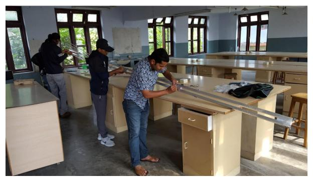
Figure 1: Mr. Suman Gautam and colleagues assembling the LPDA before mounting it on the roof of science building.
