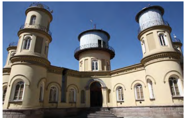
Figure 3: Building of the Quito Astronomical Observatory after the restoration in 2010.
