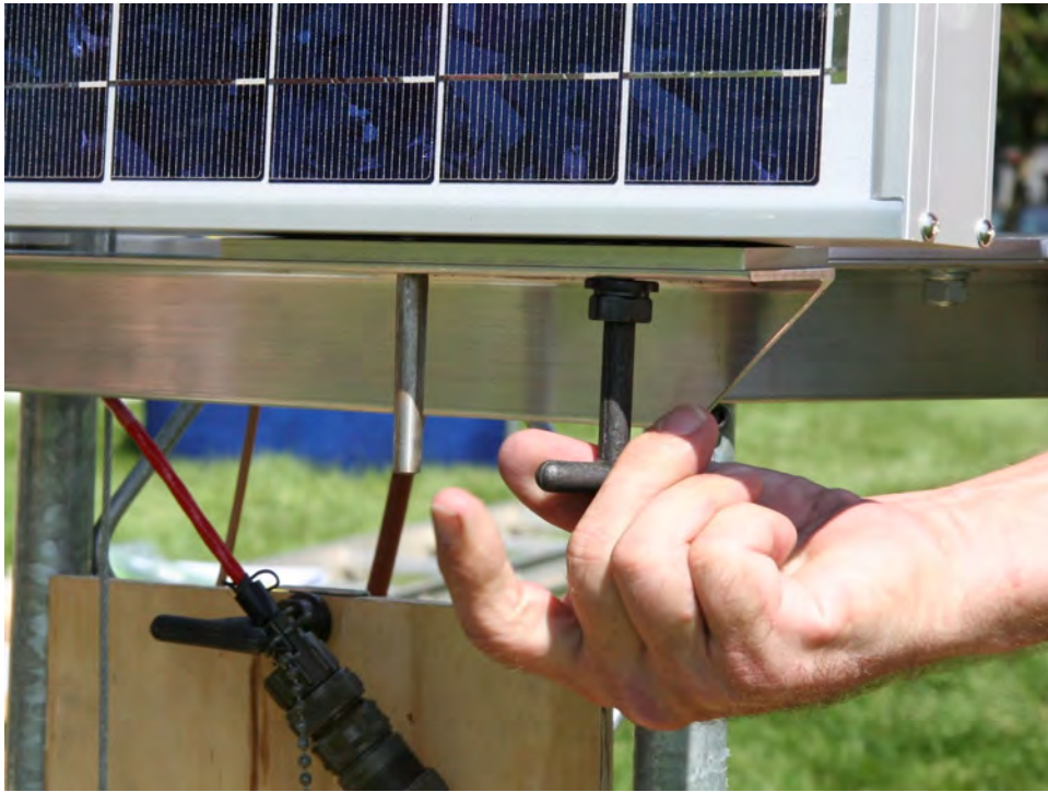
Figure 14. T-bolts used for solar panel assembly.
