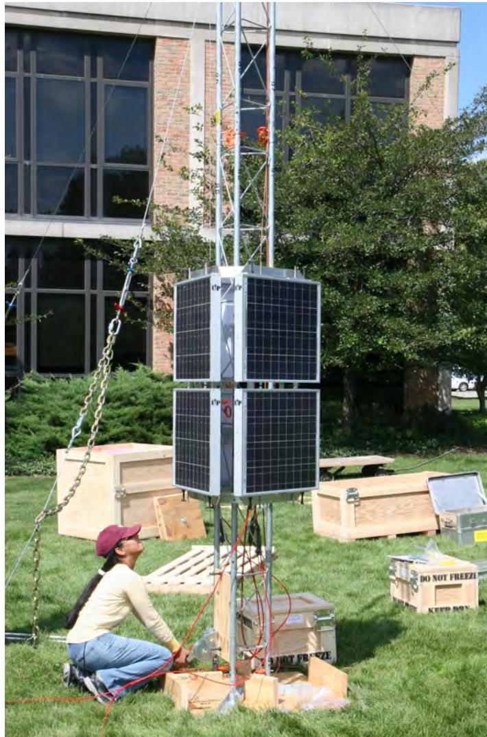
Figure 15. Winch mechanism for installation of the solar panels on the tower.
