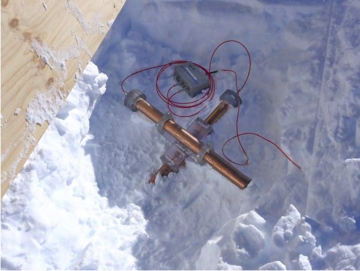
Figure 9. AAL-PIP search-coil magnetic sensor installed in a snow pit.
