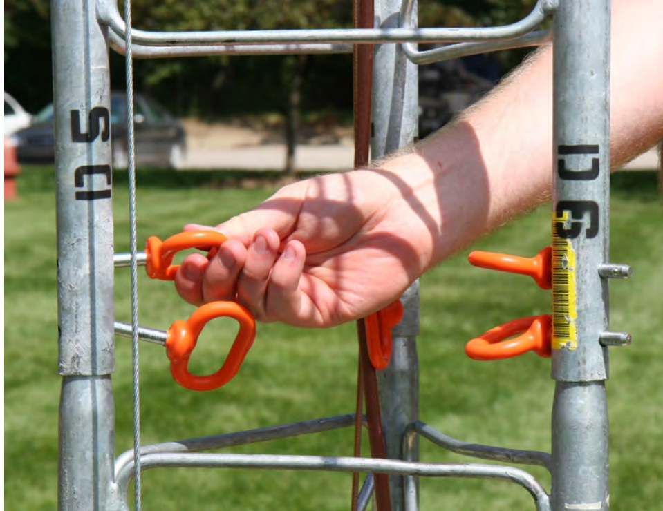
Figure 13. Pins used for tower assembly.
