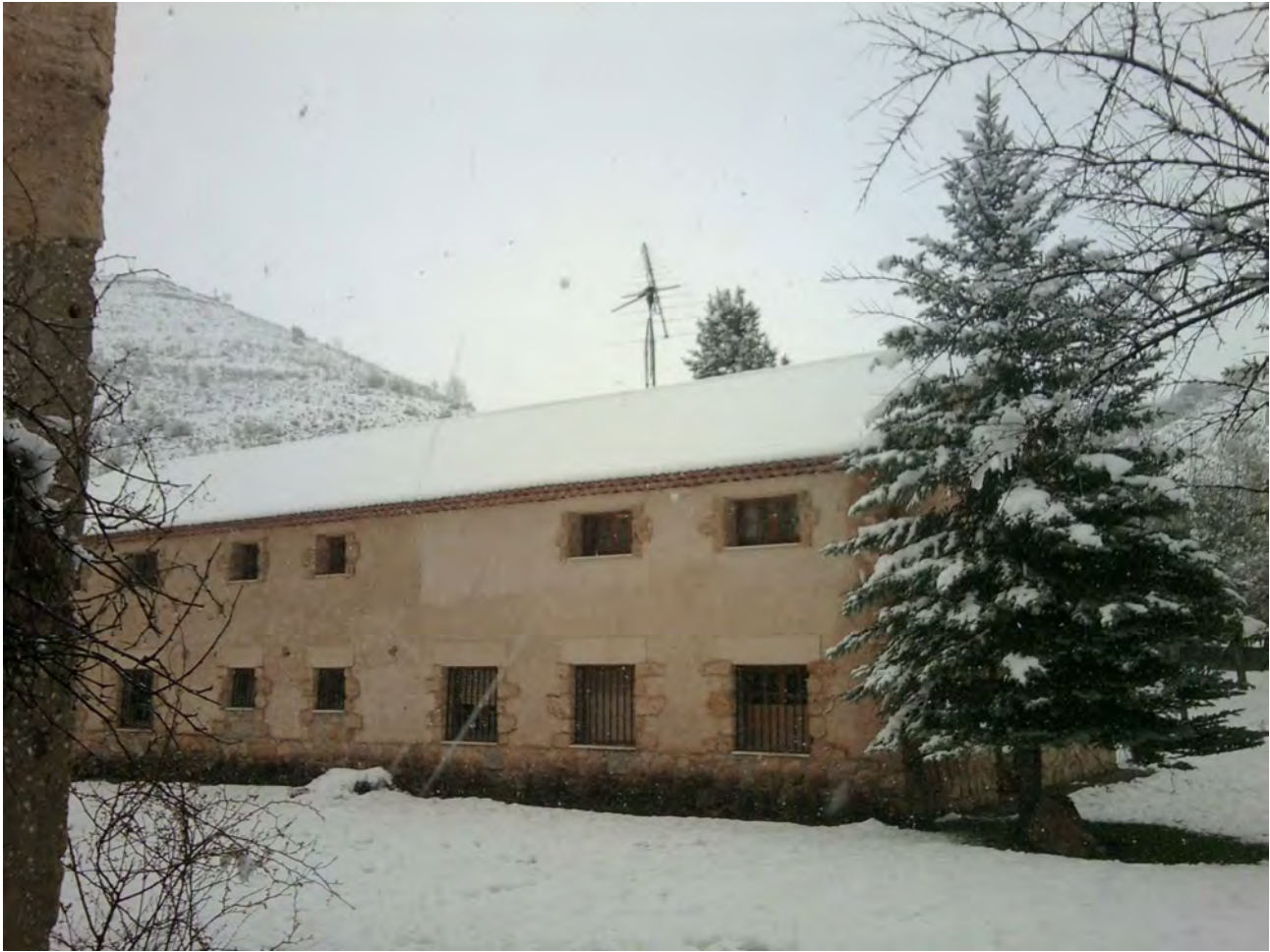
Fig 3: Log-per antenna on top of the roof with tracking system. Photo by Andrés Russu
