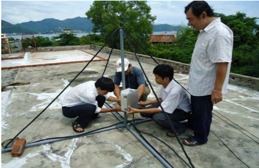
Mounting the Preamplifier Box to the VLF Antenna
