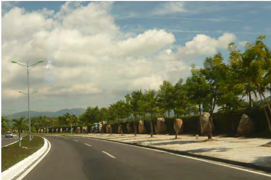
The highway from Airport to Nha Trang City
