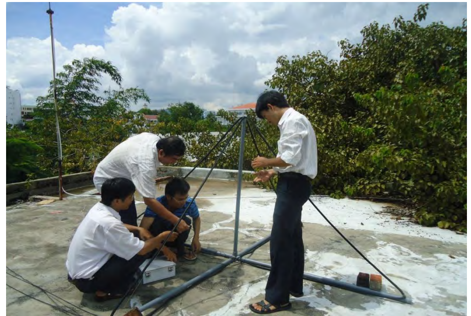
Assembly the VLF Antenna
