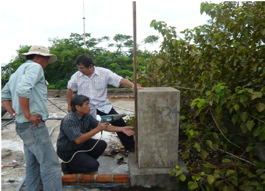
Setting up the GPS antenna on the roof of the building
