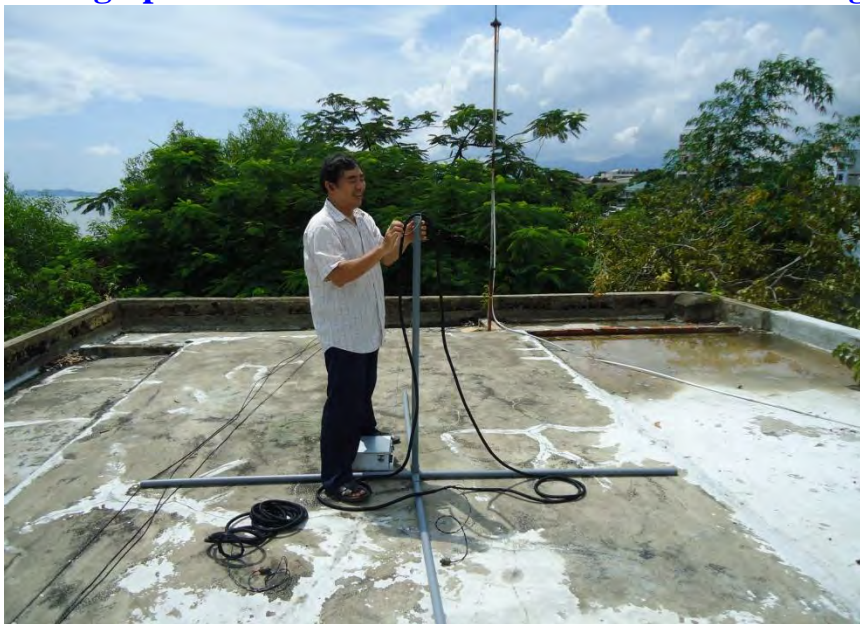
Assembly the VLF Antenna
