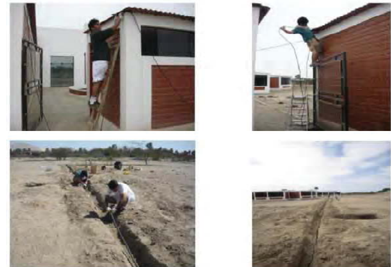
Figure 7: Cable laying process
