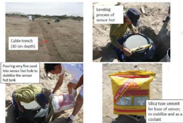
Figure 5: Works progress on sensor hut and cable trench
