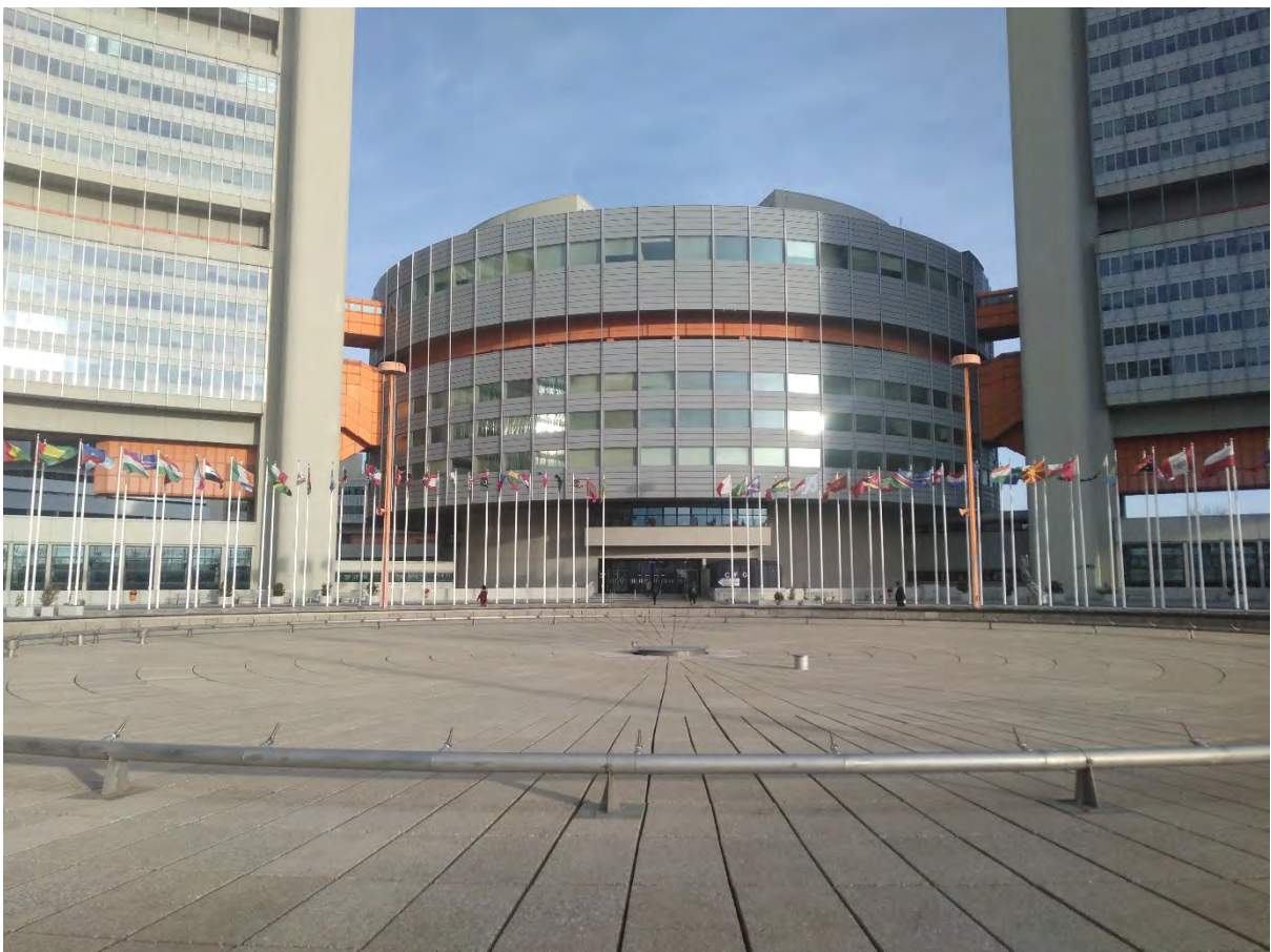
Figure 2: UN Vienna Rotunda (C-building)
