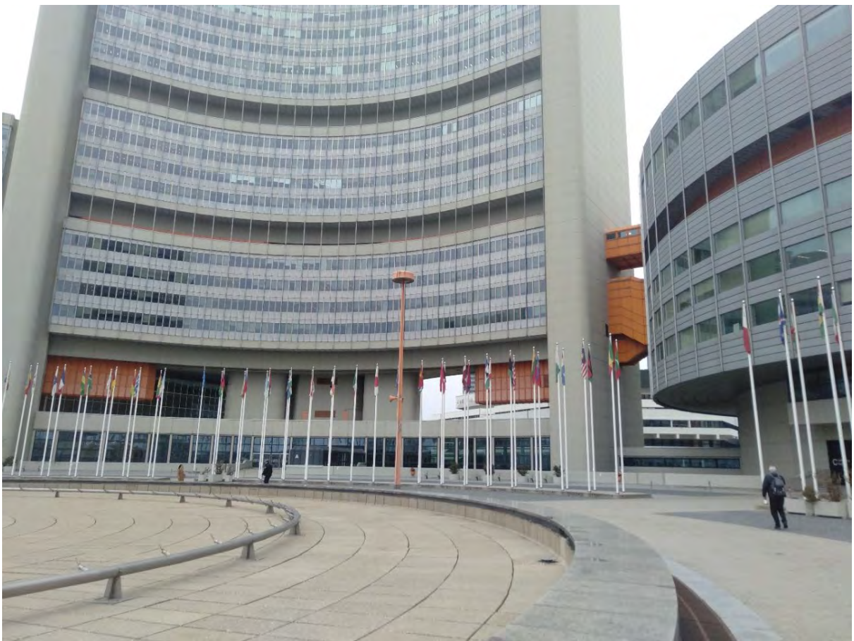
Figure 4: UN Vienna F-building
